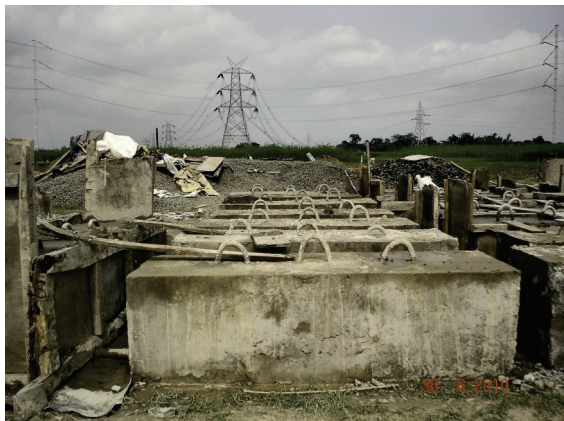
Figure 3. Concrete block anchors after fabrication on-site
