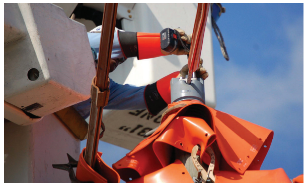
Figure 3. Example use of insulating blankets to shield sensor connector area from live line
