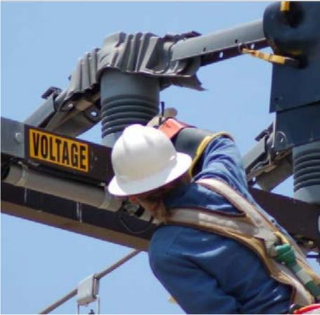
**Figure 2.** Example use of insulating blankets to shield live line from sensor connector area.
