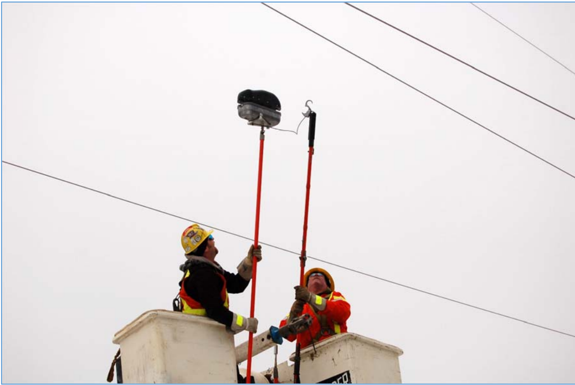
Figure 4: Next generation DLR line monitors can be installed live-line up through 765kV.
