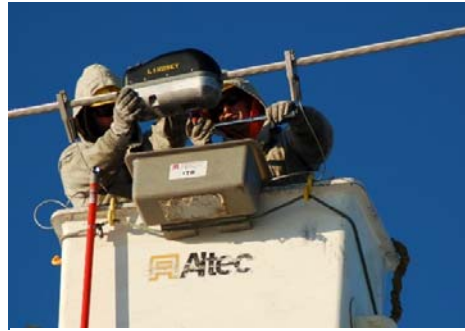
Figure 5: Live line installation of sensor
