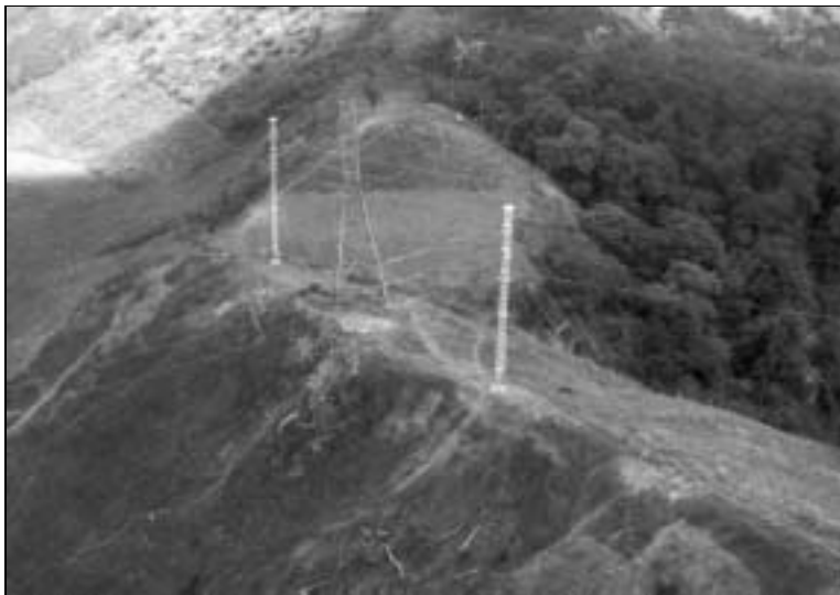
Figure 9 The photograph to the left shows the placement of the two ERS horizontal-vee structures directly on top of the ridge. Note that the dead-end insulators and hardware are in the span and to the left of the ERS in the foreground.
