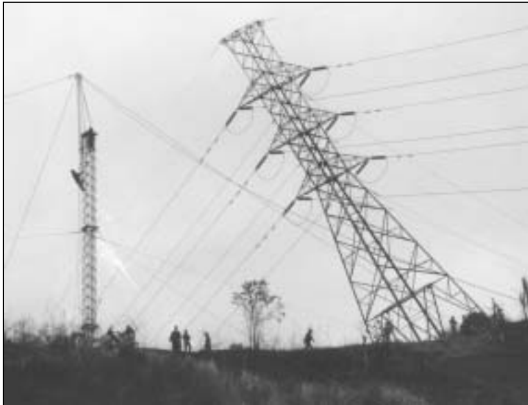
Figure 8 Vandals cut the legs of tension tower No. 44. This tower is located on the top of a narrow ridge. In order to keep the line energized, the conductor from one circuit was transferred to the ERS horizontal-vee structures while the other circuit was energized.
