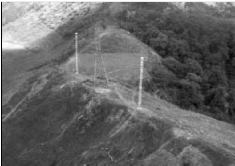
Figure 9 The photograph to the left shows the placement of the two ERS horizontal-vee structures directly on top of the ridge. Note that the dead-end insulators and hardware are in the span and to the left of the ERS in the foreground.
